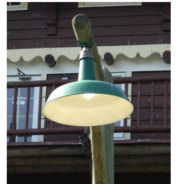
Above: This shielded light in a national park directs light downward and keeps the light out of the sky, where it can wash out the view of the stars and Milky Way.
