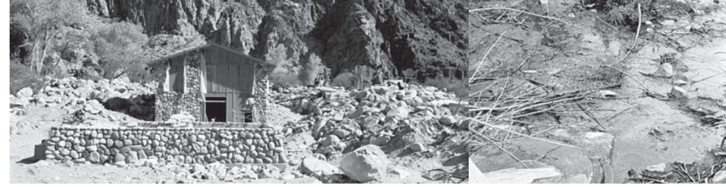
PHANTOM RANCH SEWAGE TREATMENT PLANT UNDER CONSTRUCTION: OVERVIEW - SOUTH ELEVATION. EXTERIOR. JULY 1981. NPS, HODAPP. CLOSEUP OF SEPTIC TANK SHOWING FLOW OUT OF MANHOLE. CIRCA 1981. NPS PHOTO.
