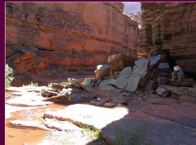
Photo of Deer Creek patio, September 2006, after a major rockfall which occurred unwitnessed sometime the previous spring. Notice the big chunks of rock, spalled off from the cliff above.
