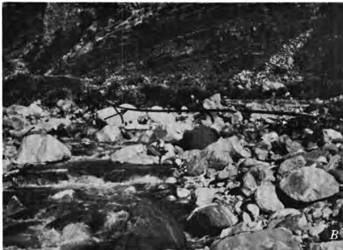
FIGURE 12.—Bright Angel Creek before and after the flood of December 1966. A , Stream channel before the flood; poles show the alignment of the pipeline (arrows). B , Exposed pipeline (arrow) after the flood.
