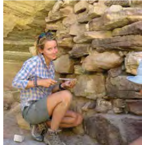
Erin Brugler at work repointing at Beamer's Cabin.
