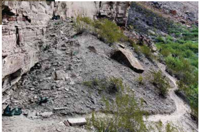
Whitmore post-work. photo: NPS
