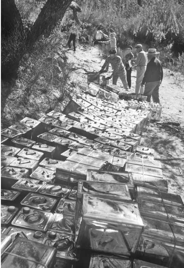
Gas supply at Lees Ferry NAU. Pht. 96.4.94.15 Bill Belknap photo.
