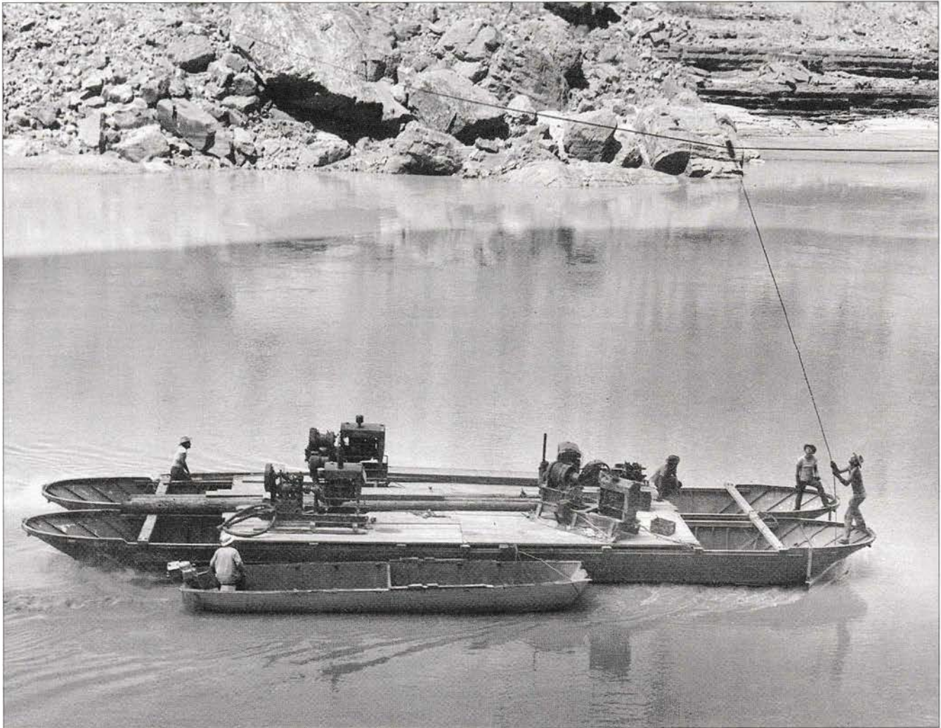
Drilling barge being moved
