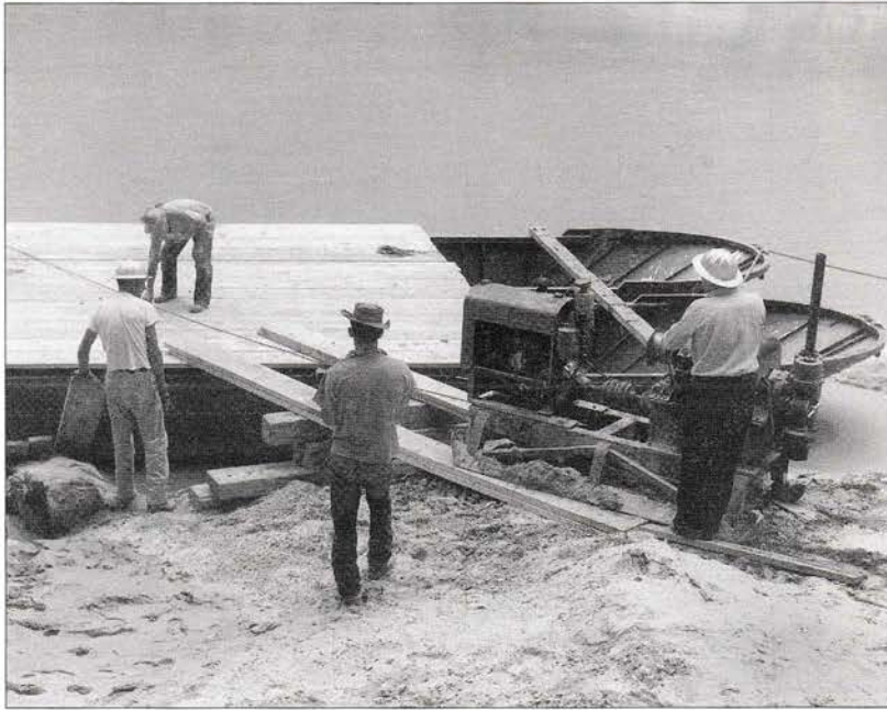
Crew moving drilling machine onto barge
